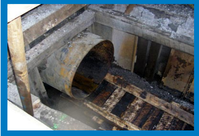
The host pipe was accessed through excavated pits.
