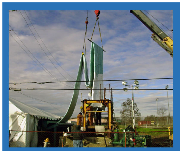
A crane positioned the impregnated felt over the hole.
