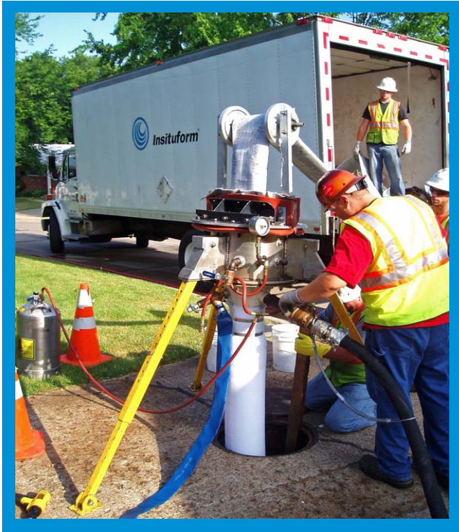
Resin-impregnated liners were shipped under controlled conditions to designated installation points.
