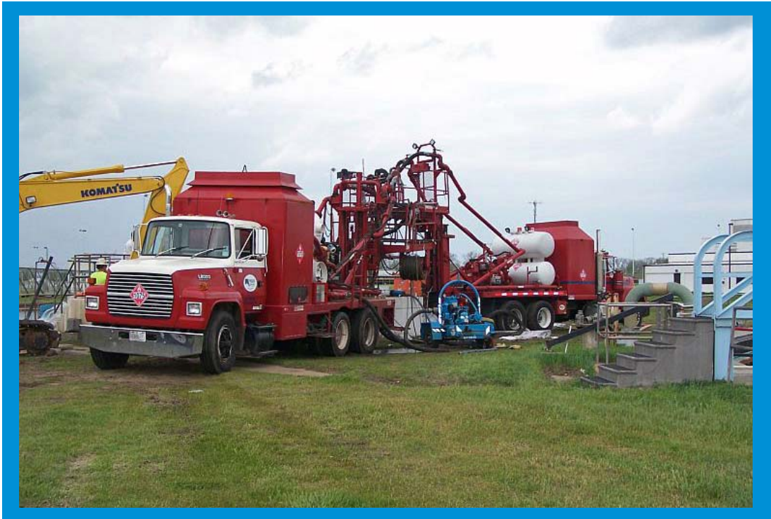
To minimize clarifier downtime, heated water from two boiler trucks accelerated resin cure.
