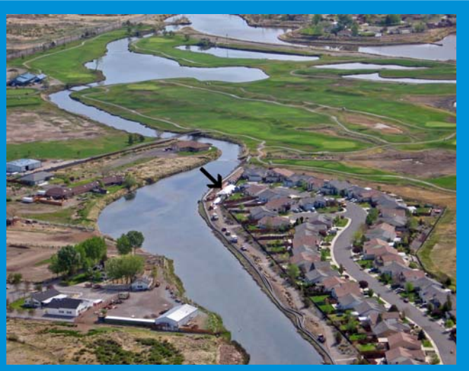
CIPP preserved the scenic Rosewood Hills area. The arrow points to the location of the on-site wet-out facility.
