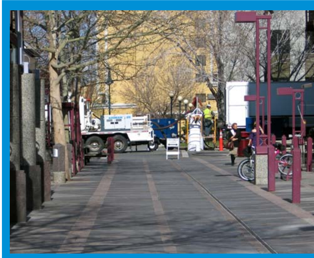
Trenchless technology for downtown Reno prevented disruptions to the city's busy convention trade.
