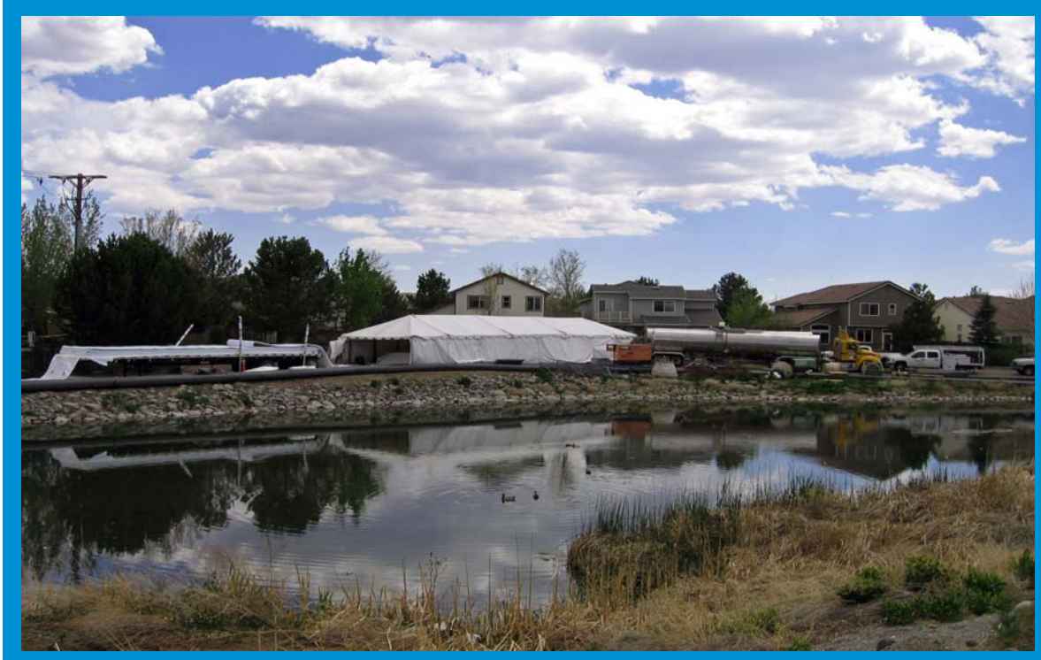
Over-the-hole insertions at existing manhole sites eliminated the need for trenches.
