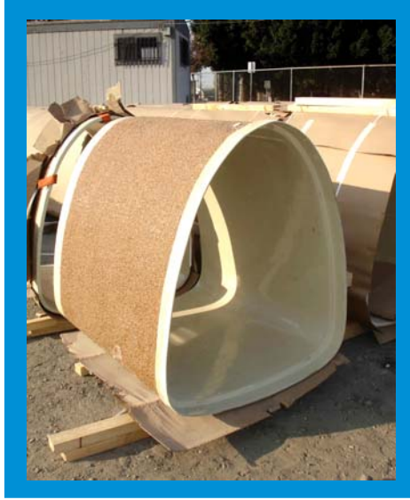
The new composite liner panels conform to the semi-elliptical shape of the host pipe
