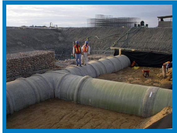
Integral ribs allow the buried portion of the intake pipe to withstand heavy loads.
