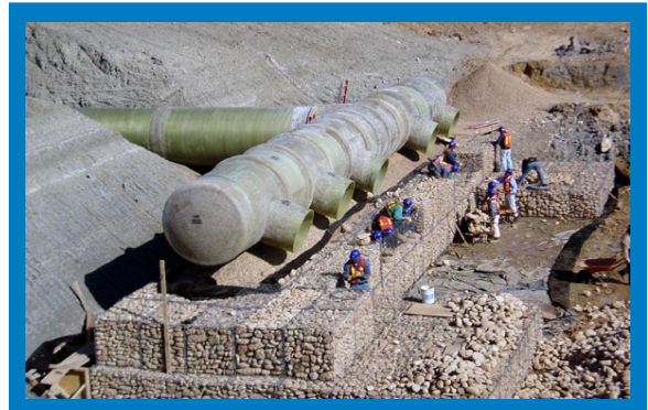
Workers install the composite diffuser for the seawater intake pipe.
