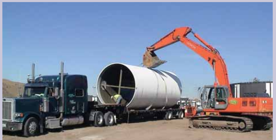
Low weight eases installation of the Denver sewer pipe.
