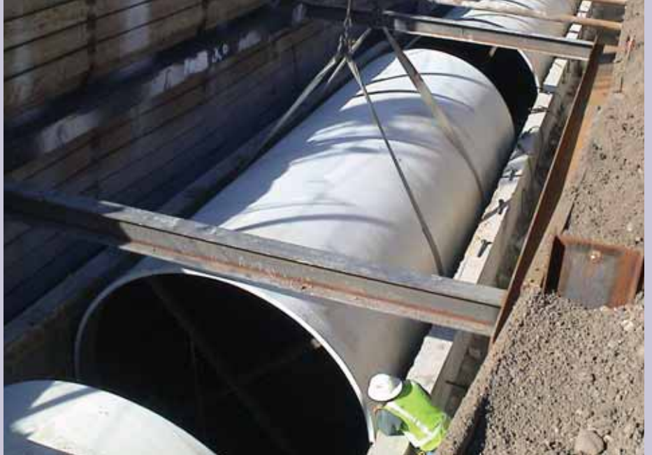
Denver sewer pipe installed in bottom portion of concrete culvert.
