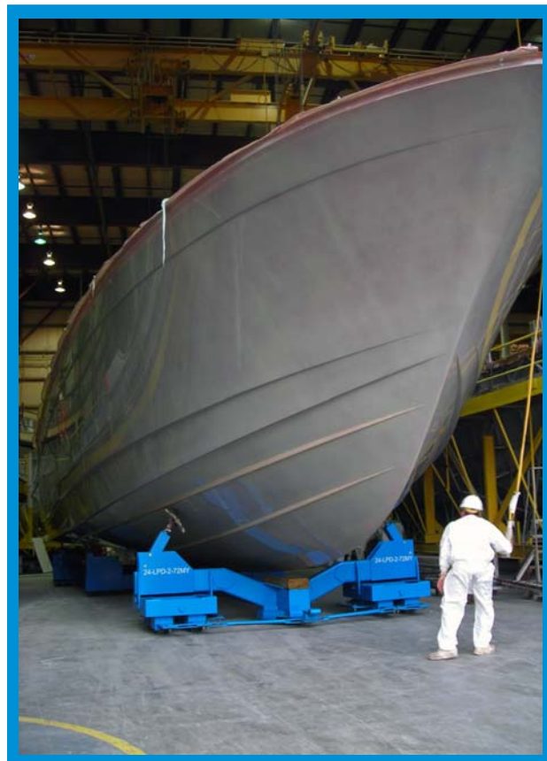
Using a clear gel coat allows the finished hull to be inspected after it is pulled from the mold and before an exterior marine coating is applied.
