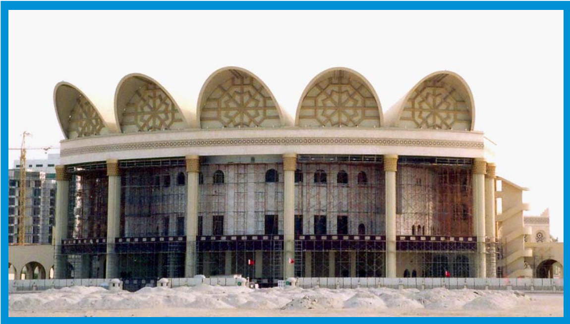
The five vaults are 92 feet (28 meters) above ground level.
