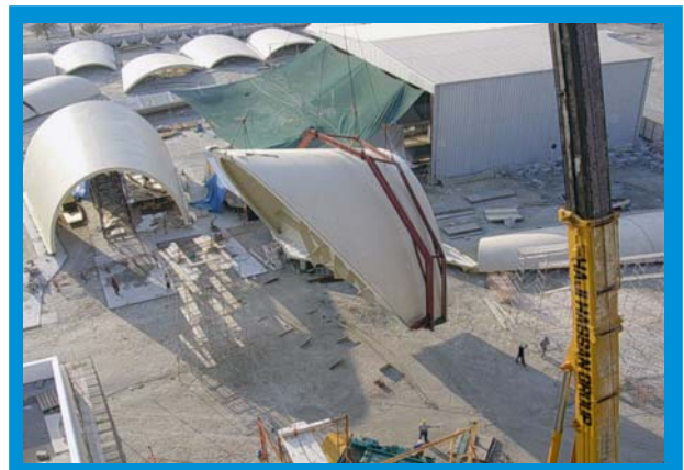
A front section is crane-lifted for installation atop the Conference Hall.
