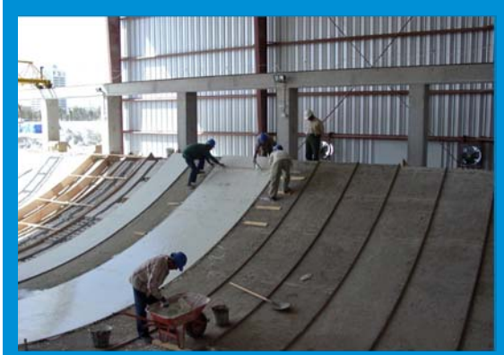
Molds were built of reinforced concrete and finished with a cultured marble surface.
