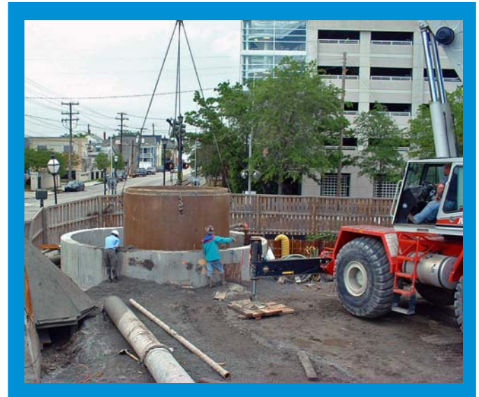
The huge polymer concrete structures were installed in “stack-up” sections.
