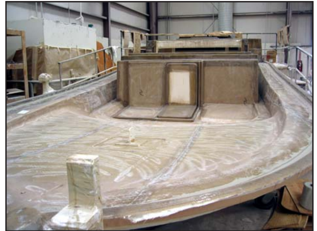
The surface of the deck-in-progress is mechanically ground to ensure good adhesion of the next layer of composite laminate.
