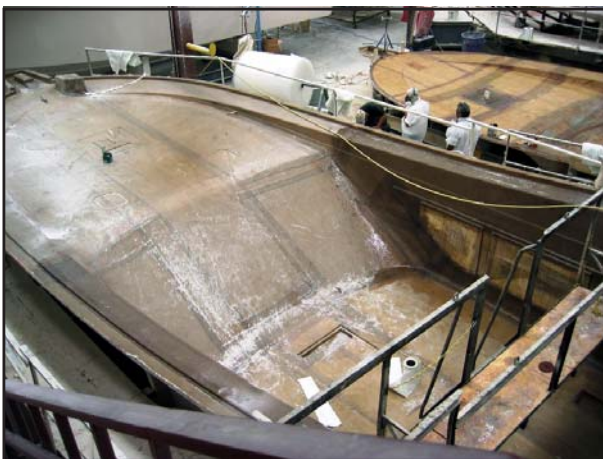
Cabo Yacht decks are handcrafted of fiberglass roll goods and AOC resin by highly skilled workmen.
