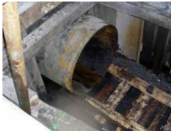
The host pipe was accessed through excavated pits.
