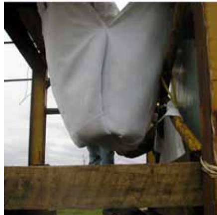
The felt tube was secured to a frame over the hole (top) prior to inversion (bottom).
