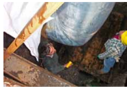
The tube was inverted through the host pipe.
