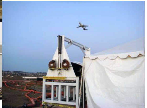
CIPP eliminated the need for pipe excavation and replacement.
