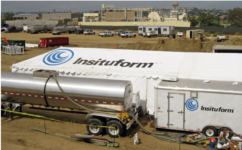
Vipel® technology was used for a custom composite liner.
