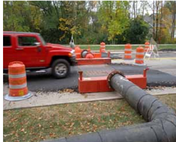
By-passes were smooth enough to allow 25 mph traffic.
