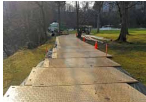
Access matting helped workers reach the job site and protected the terrain during repair.
