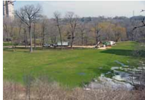
The rehabilitated pipe and culvert carry storm water through a golf course.
