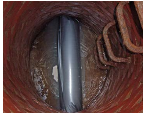
The fiberglass liner was inflated on top of the slip sheet.
