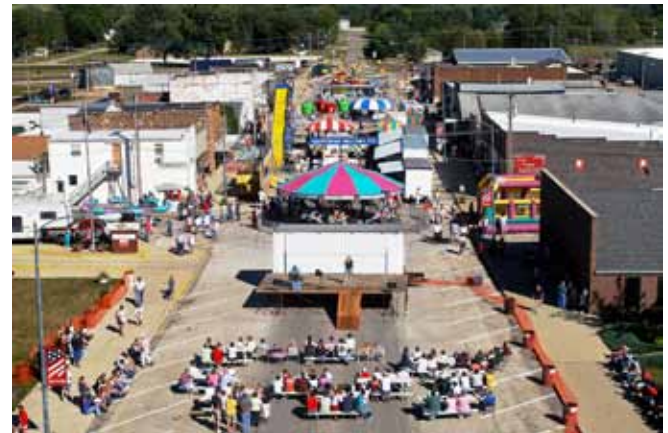
With trenchless CIPP upgrading the sewer's underground, the Southern charm on Collierville streets was not impacted.
