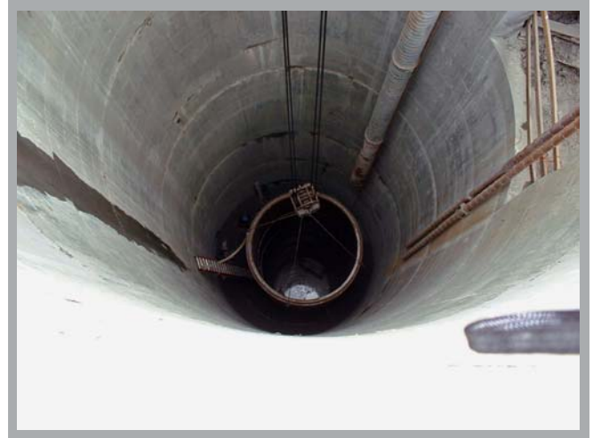
The average depth of a completed shaft was 80 vertical feet.
