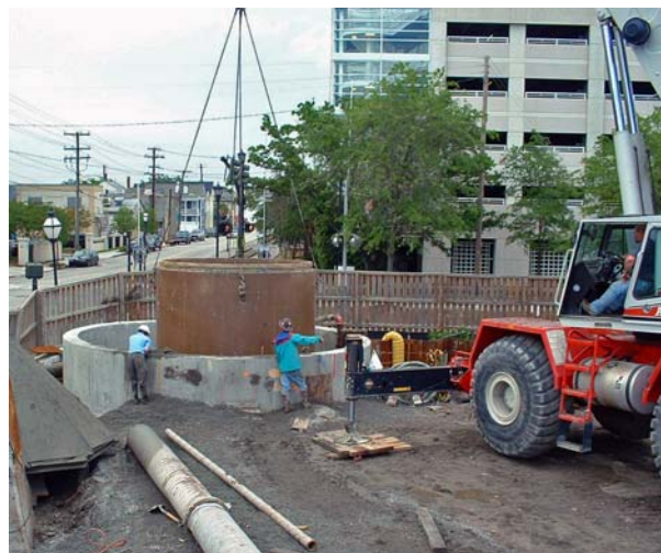
The section is lowered into the shaft.
