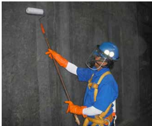
The Vipel® resin formulation addressed thixotropic needs for vertical application.
