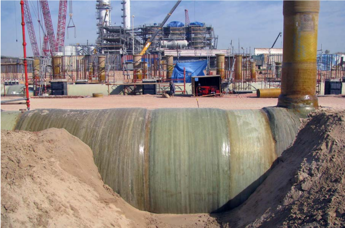
Vipel® technology joins cooling water pipeline for the world's largest HDPE plant.
