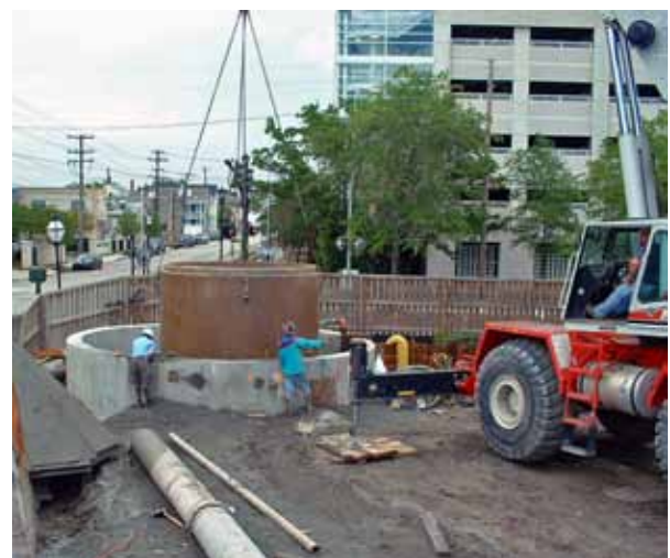
The section is lowered into the shaft.
