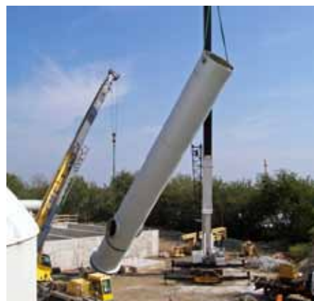
Two 72-foot tall stacks were installed.
