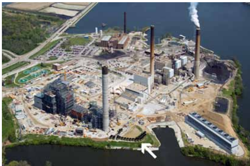
In this aerial view of the project site, an arrow points out the composite liners ready to be installed in the new stack.
