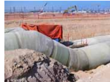
The project included elbows and connectors for above- and below-ground pipe
