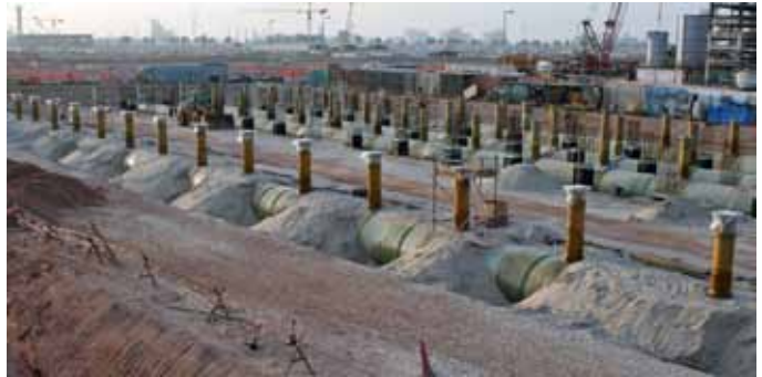
More than 850 joints were formed in 12 months time.
