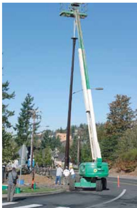
The lightweight DuraPole utility pole is easily lifted in place.
