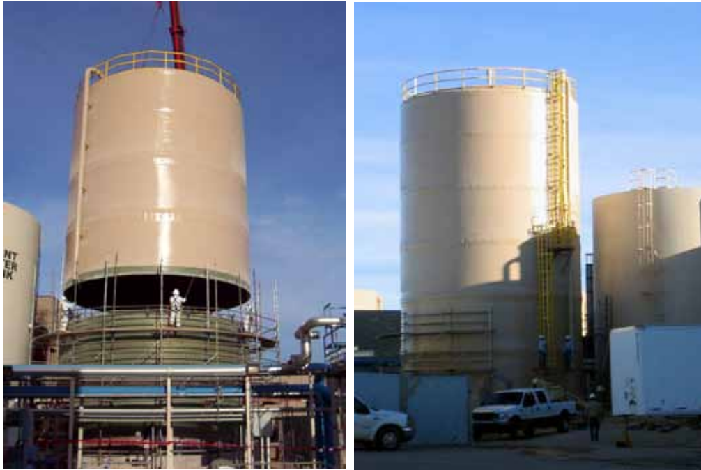
The completed 350,000-gallon tank withstands three potable water rinse cycles a day.
