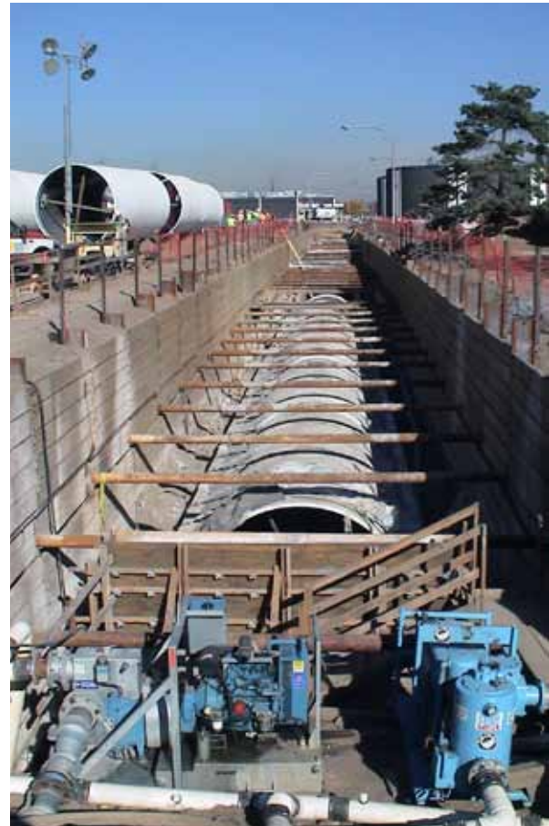
Five hundred feet of composite pipe were installed.
