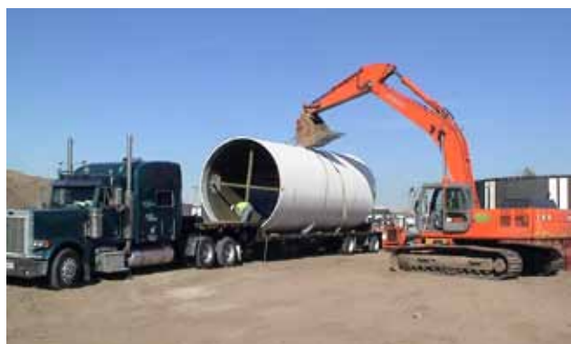
Lightweight composite pipe is easily moved with less expensive equipment.
