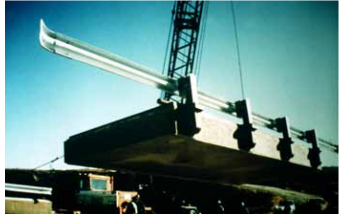
KSCI manufactures composite bridge components with AOC's Vipel® F701 Isophthalic Polyester resin.
