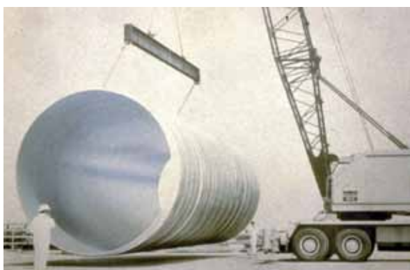
These water pipes, installed in 1978, were ordered by the Jacksonville, FL Electric Authority. They were ordered to carry warm water out of the power plant into the Atlantic Ocean, and they have a minimal effect on marine life.
