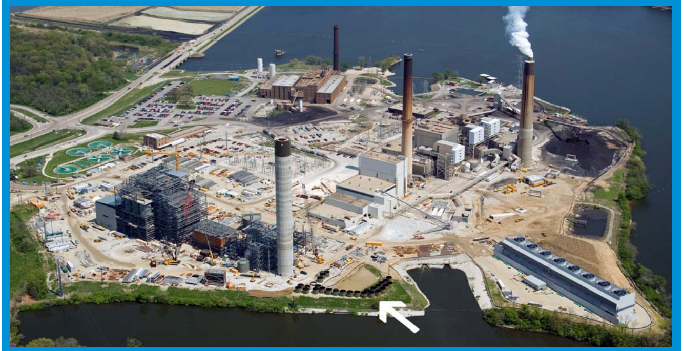
In this aerial view of the project site, an arrow points out the composite liners ready to be installed in the new stack.
