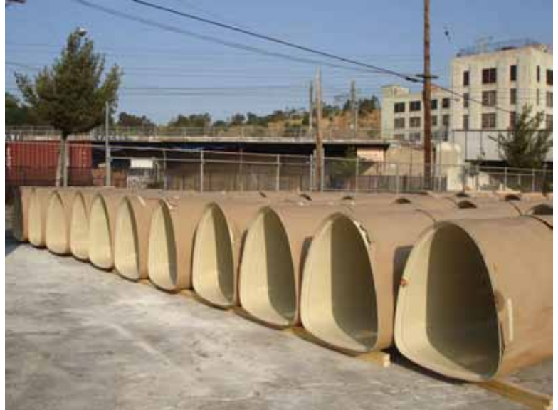
The composite panels were shipped to the Los Angeles job site and installed in a matter of weeks
