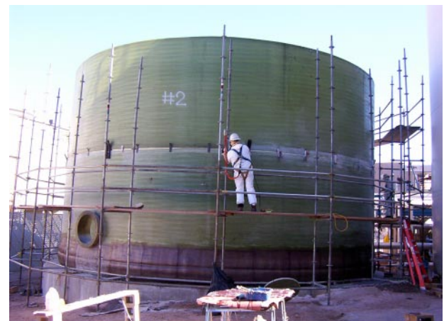
Tank sections were assembled and bonded to each other at the nutritional products manufacturing plant.
