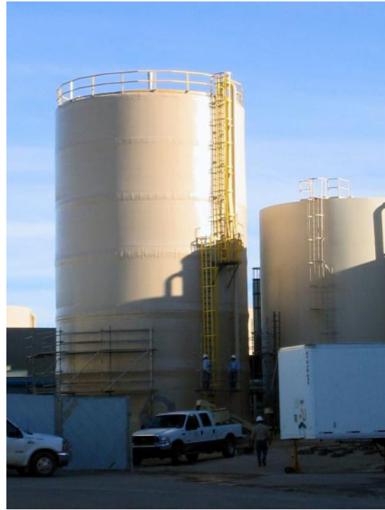
The completed 350,000-gallon tank withstands three potable water rinse cycles a day.
