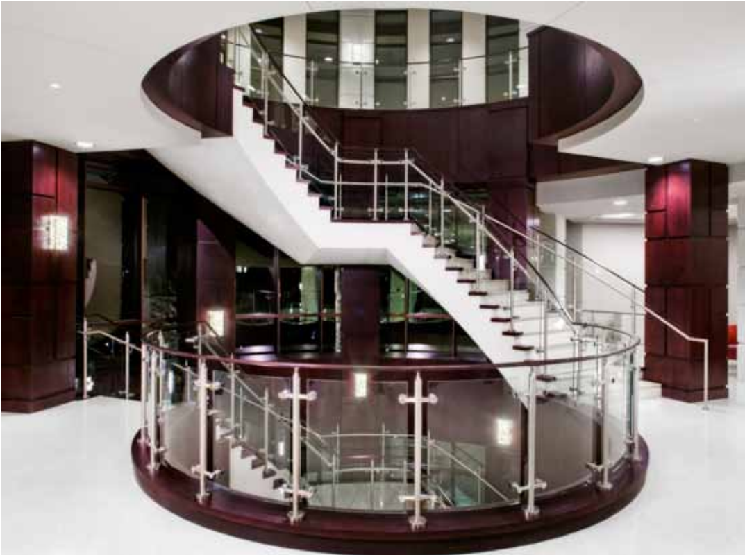
Composite forms gave this dramatic staircase its shape.
