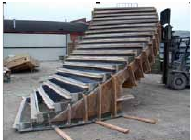
Section ready for delivery
