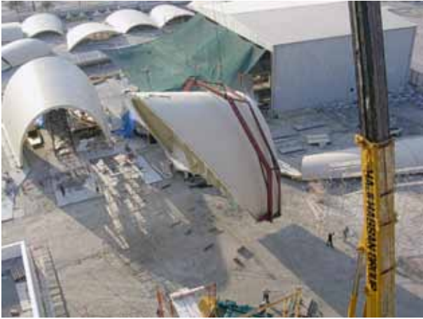
A front section is crane-lifted for installation atop the Conference Hall.
