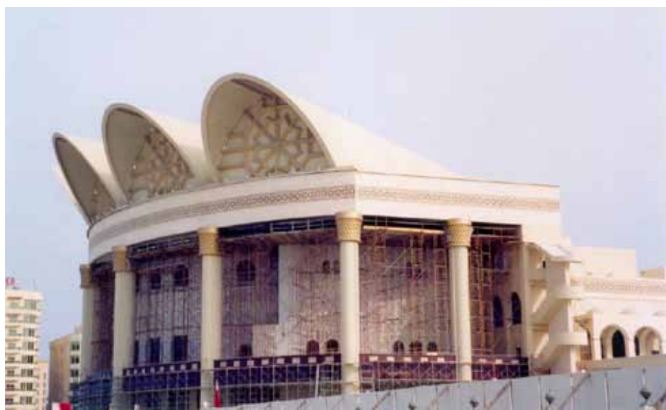
The five vaults are 92 feet (28 meters) above ground level.
