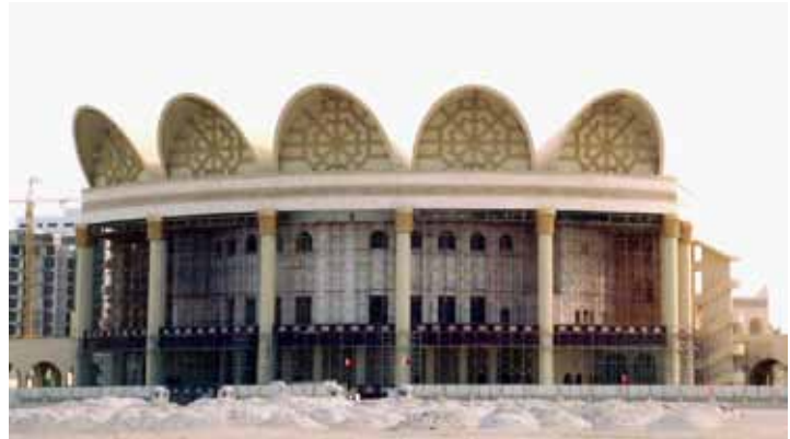
The half-cone-shaped vaults taper from 52.5 by 30 feet (16 by 9.25 meter) dimensions in front to 26.2 by 19.7 feet (8 by 6 meters) at the rear.
