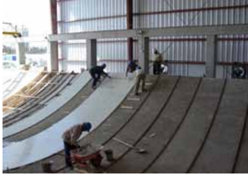
Molds were built of reinforced concrete and finished with a cultured marble surface.
