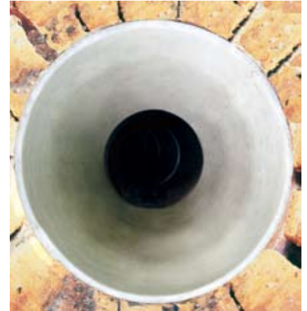
After repair with Vipel® technology
