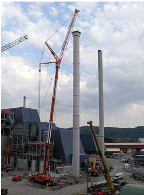
The composite liners were installed in a combined steel housing that was shipped to the plant site.
