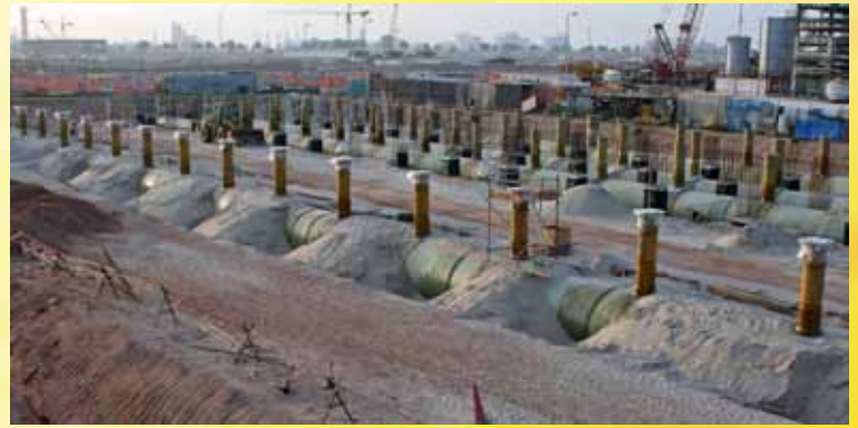
Vayyu crews field-laminated 858 joints.
