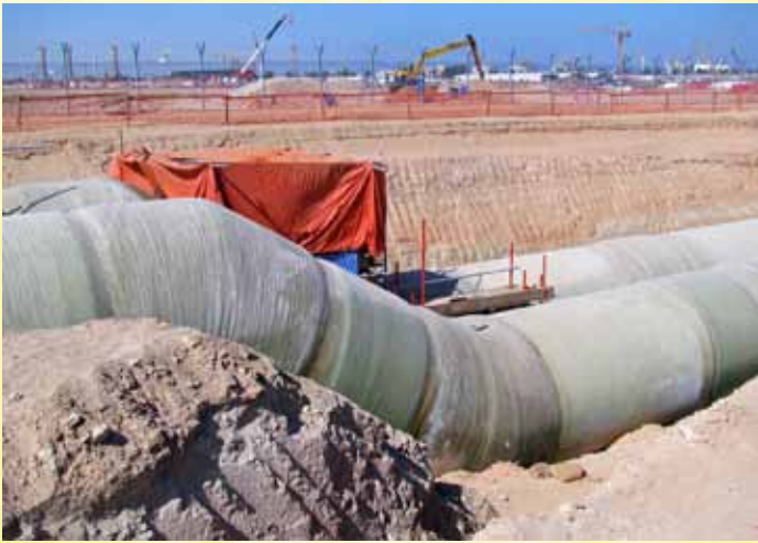
The job involved above- and below-ground pipe.
