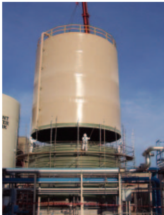
Figure 3. A composite rinse tank for processing nutritional products is installed.
