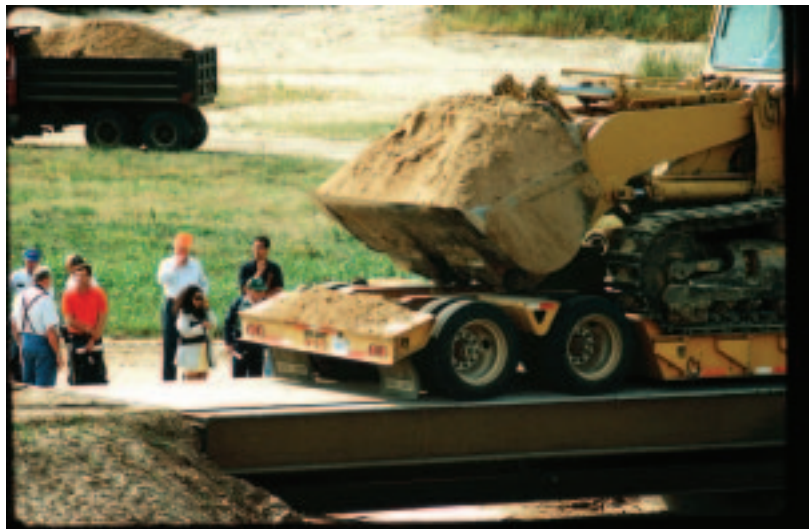
Figure 7. A short-span composite bridge is load-tested shortly after its installation in 1994. The bridge is still in service today.
