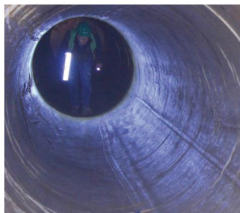
*Adrian Cordero, an engineer with Tubepol, inspects a rehabilitated pipe under the Mexico-Tuxpan Highway.*
