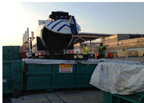
*Clean Water Works removed debris from the sewers prior to installing CIPP liners.*
