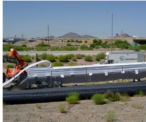
*To repair large diameter concrete pipe, new liners were created by impregnating miles of Insituform® felt with Vipel resin. (Image is used courtesy of Insituform Technologies, Inc.)*
