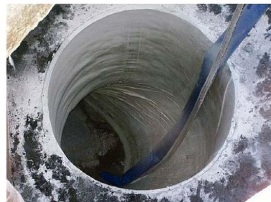
*After the splitter box discharges were cleaned and prepared (left), they were lined with CIPP (right) and sealed.*
