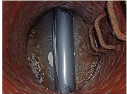
*The fiberglass liner was inflated on top of the slip sheet.*
