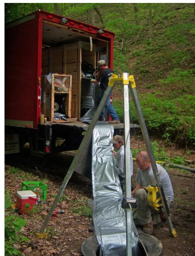
*To eliminate excavation, the special Blue-Tek® slip sheet was guided into the host pipe through an existing manhole*
