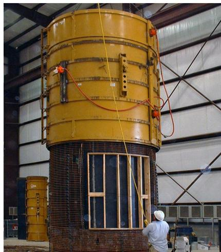
*A worker sets the formwork for casting the 12-foot high vortex section.*
