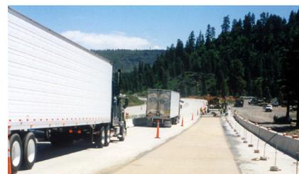
*The traffic lane can be re-opened for traffic within four hours of the polyester concrete application.*
