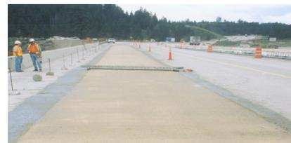
*The surface is cleaned and primed prior to application of the polyester concrete.*
