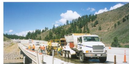
*New polyester concrete deck overlays are being applied to multiple bridges on Interstate 80 between the California towns of Truckee and Floriston.*
