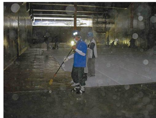
*More than 40,000 square feet (3,700 square meters) of concrete surface were rehabilitated and strengthened.*
