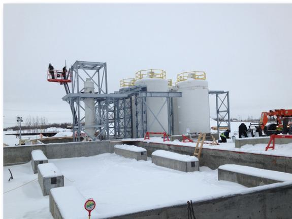
*Construction on an HCL transload facility in Alberta, Canada, included these four surge capacity tanks and scrubber (left), all of which feature Vipal® corrosion-resistant resins.*
