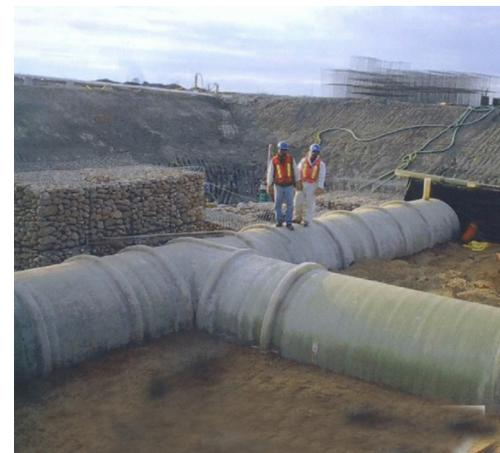
*Integral ribs allow the buried portion of the intake pipe to withstand heavy loads.*
