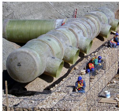
*Workers install the composite diffuser for the seawater intake pipe.*
