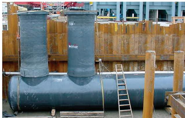
Beetle Florida uses AOC's Vipel F737 resin to filament wind pipe for the cooling water system of a new, 1,186 megawatt generating facility of PSEG Power LLC. The natural gas-powered facility is being built next to an existing plant that will be retired when the new project is complete in 2003.
