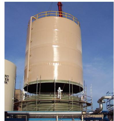
The completed 350,000-gallon tank withstands three potable water rinse cycles a day.
