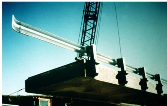
*KSCI manufactures composite bridge components with AOC's Vipel<sup>®</sup> F701 Isophthalic Polyester resin.*
